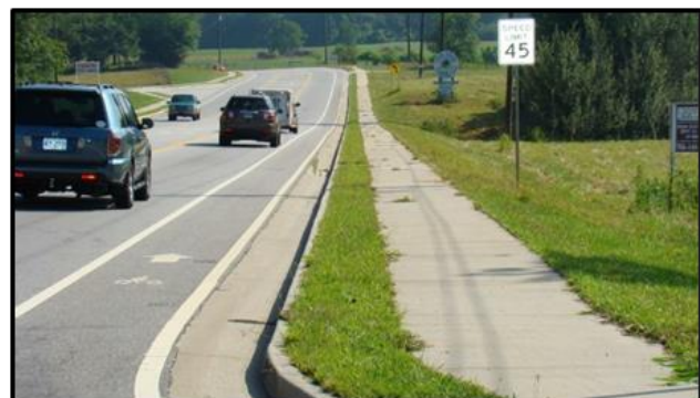
Figure 7. Bike Lanes and Sidewalks along GA Hwy 75
