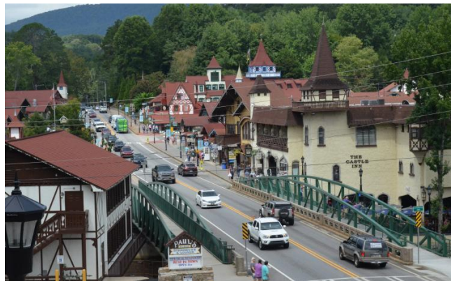
Figure 8. Pedestrian Bridge in Helen
